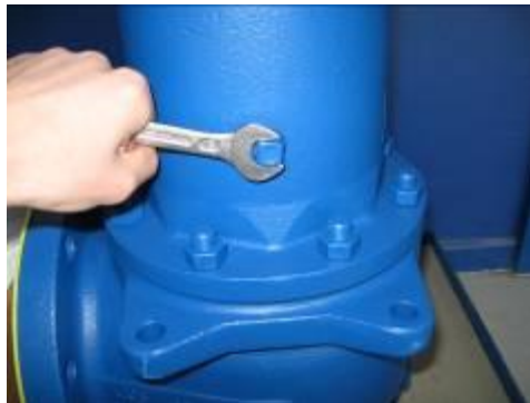
Fig. 2 Sealing the drain hole
