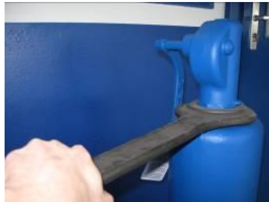
Fig. 3 Installation of the lever and cap
