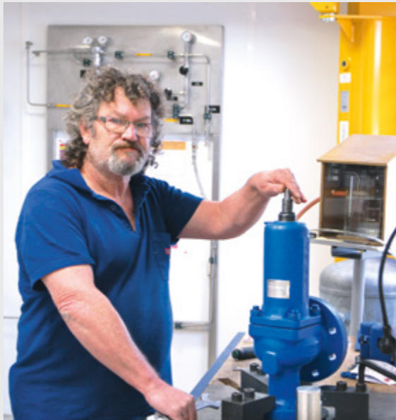
Local valve adjustment at the central warehouse in Toulouse
