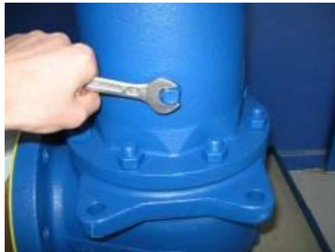
Fig. 2 Dealing the drain hole
